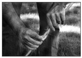
Step #6 Remove the come-a-long and the Chicago grips from the strand. Finish installing both legs of the GUY-LOCK. Ensure that all rod ends are completely snapped in place.
