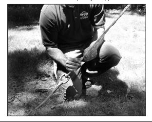
Step #6 Next, remove the come-a-long and Chicago grips from the strand. Finish installing the first leg of the GUY-LOCK. Ensure that the rod ends are completely snapped in.
