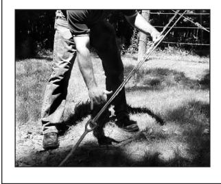
**Step #3** Wrap a leg of the GUY-LOCK on the main down guy installing at least 2-3 pitches.
