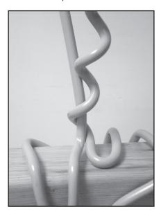
Step #5 Repeat Steps 1 - 4 to install the second deterrent. Make sure that the middle uprights are close enough to complete the application in Steps 7 and 8. Also note that the helical upright must be next to a straight upright to lock them together.
