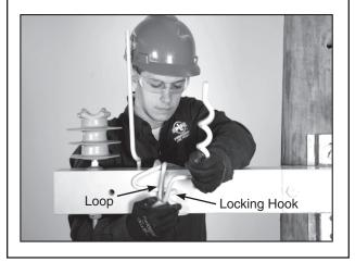
Step #6 Lock in the second deterrent using the same procedures as shown in Steps 3 and 4. Make sure it is close enough to the first BIRD PERCH DETERRENT crossarm to lock them together.
