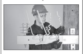
Step #4 Lock the other loop of the second upright of the BIRD PERCH DETERRENT into the Locking Hook on the other side of the crossarm. Once both sides are locked, the unit will not slide on the crossarm. Ensure proper location prior to locking into place.
