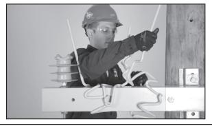
Step #8 Wrap the helical upright all the way to the top until it snaps in position.
