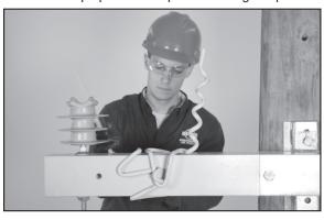
Step #7 Wrap the helical upright of the second deterrent around the straight upright of the first deterrent. Ensure that the bottom helical wrap is installed as shown below.
