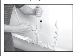
Step #6 Wrap the helical upright of the second deterrent around the straight upright of the first deterrent. Ensure the bottom of the helical upright is started on the straight upright as shown in the inset picture.
