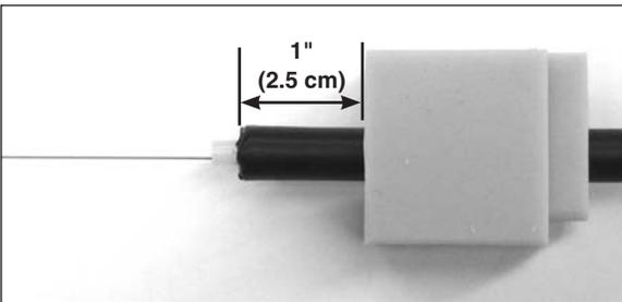
**Step #33** Wrap the felt around the drop cable as shown below.
