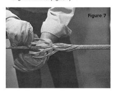
7. Snap in ends of subsets to complete the application. Repeat on the other side of the Splice Shunt. NOTE: Splitting the legs of each subset, if necessary, is permitted for easier application. (Figure 8)
