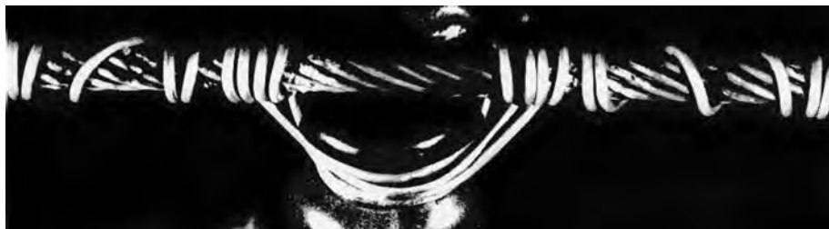
Abrasive wear on armor rods under loose tie wire.
