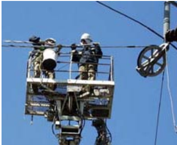
Field Trial of THERMOLIGN Formed-Wire Dead-end at a Midwest Utility
