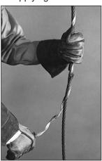
Step #7 Snap on the end of first element with thumb pressure.
