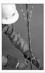
**Step #14** Snap on the two ends with thumb pressure.
