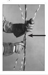
Step #12 Wrap the third element around the upper rope one or two complete turns only. Repeat on the bottom rope.
