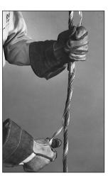
Step #10 Wrap the second element around the upper rope one or two complete turns only.
