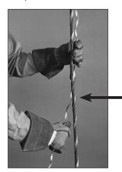
Step #9 Wrap the second element around the bottom rope one or two complete turns only.
