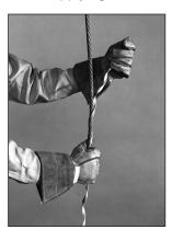
**Step #4** Snap on the end of the first element with thumb pressure.
