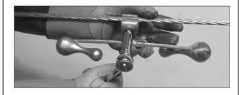
Step #3 Center the damper at the proper distance (a tolerance of 2 inches is allowed) and tighten the bolt according to the torque recommendations provided on the back of these instructions. Note: If shear head bolts have been provided, just tighten until the bolt head shears off.
