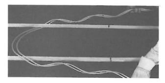
Position the first subset with the loop held AWAY from you as shown. Notice that the loop extends <u>over</u> one conductor and <u>under the other conductor</u>.
