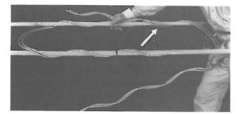
4. Position the second subset with the loop held toward you as shown. IMPORTANT: again notice that the loop extends <u>over</u> one conductor and <u>under</u> the other, BUT <u>in reverse positioning to the loop of the first</u> subset (see figure 1).
