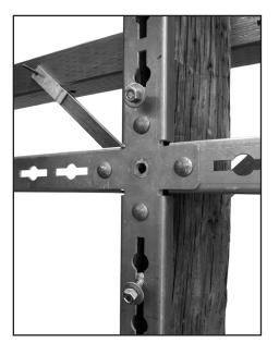
**Step #4** Hang the End Plate Bracket onto the lower carriage bolt and secure the lower bolt.
