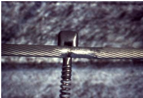
Figure 4 – Abrasion Damage at Spacer
